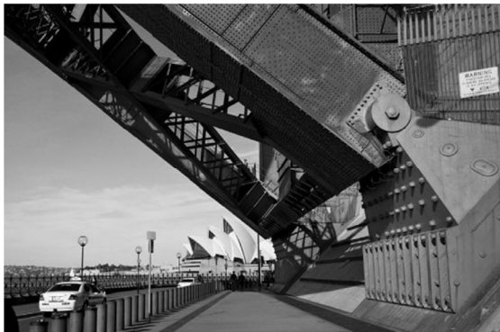
Sydney Harbour Bridge
