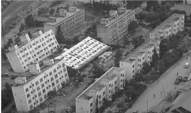
Liquefaction (Niigata, Japan 1964)
