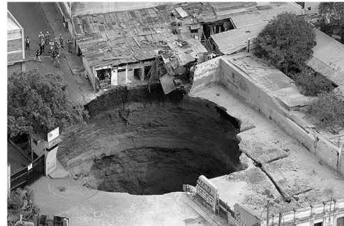
Subsidence (Pierces, Guatemala)
