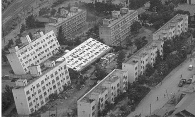
Liquefaction (Niigata, Japan 1964)
