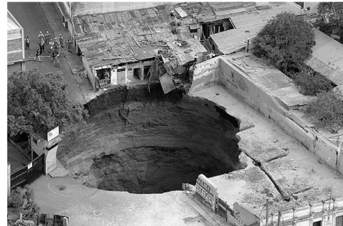
Subsidence (Pierces, Guatemala)
