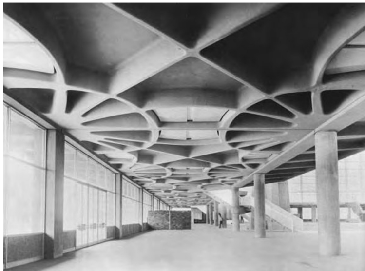
Pier Luigi Nervi, Palace of Labor Floor System Palace of Labor (Palazzo del Lavoro)
