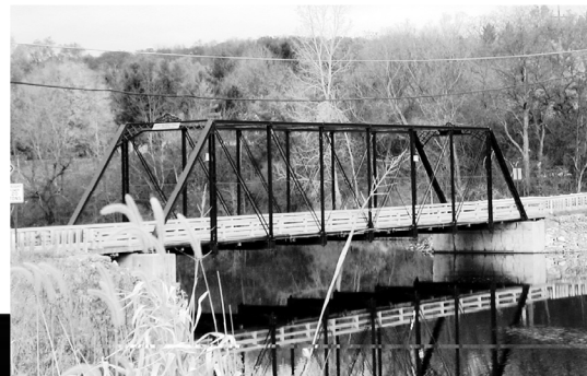
Foster Bridge, 1889 Ann Arbor, Michigan
