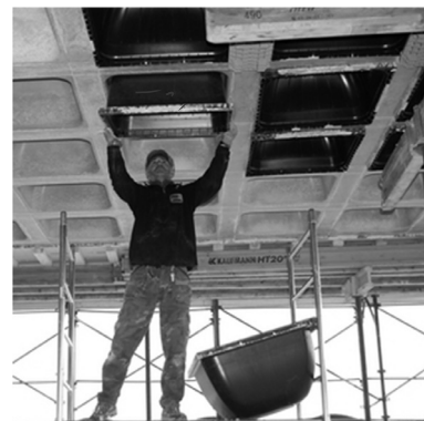
two-way waffle slab
