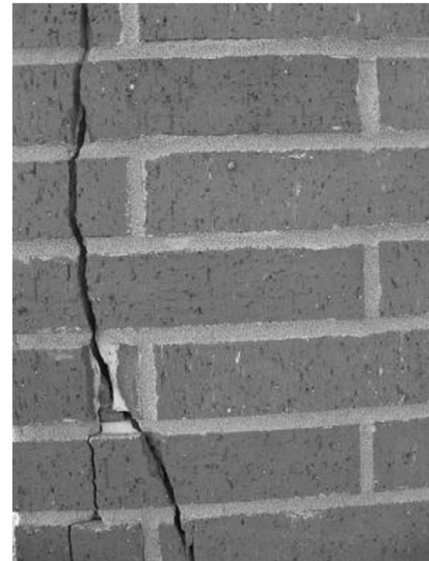
Crack due to thermal stress
