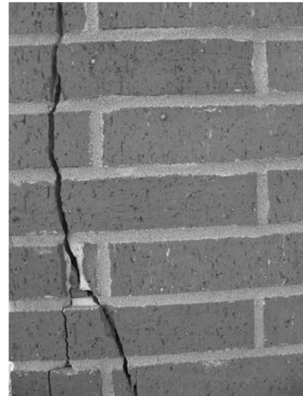
Crack due to thermal stress
